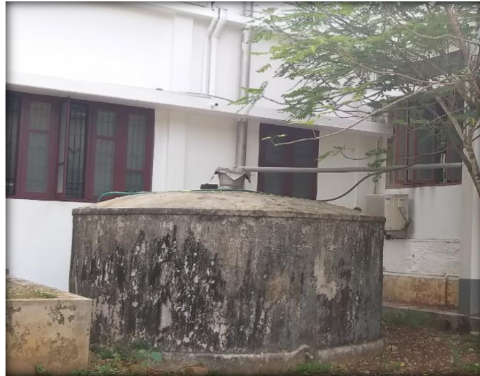
Rain Water Collected in Tank and Used in Chemistry Lab
