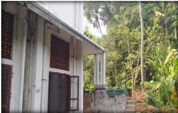
Rain Water Collected in Tank and Used in Chemistry Lab
