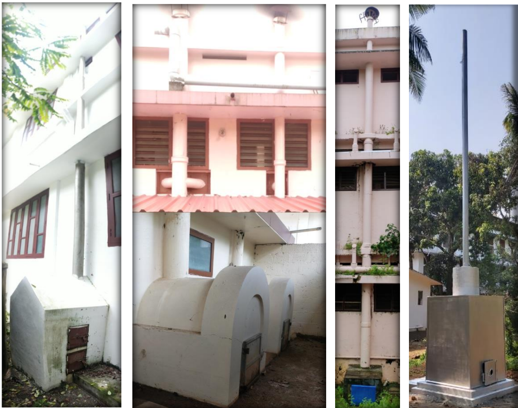
Incinerators & Waste Burning Plant
