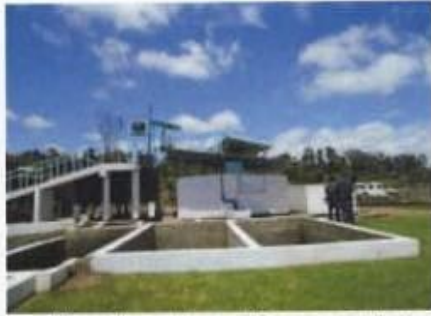
Simple systems for converting slaughter-house wastes to energy thro' High Performance (2-stage) Biogas technology. Can be turned to electricity as well. Storage in 3-ply balloons. Photos from a small town nearby to Nairobi, Kenya, East Africa. Courtesy: UNIDO
