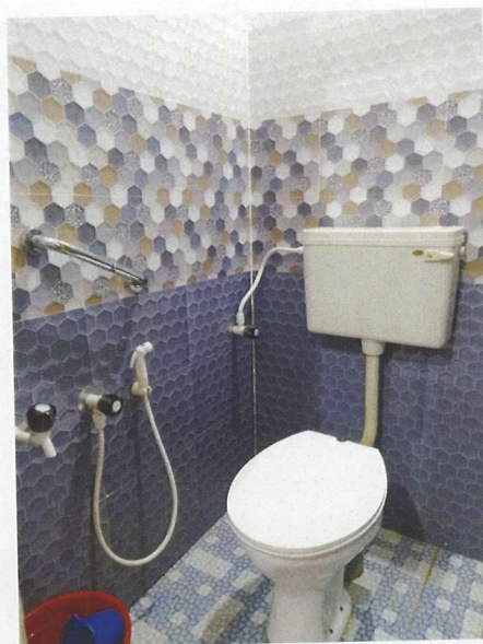
One of the accessible toilets at Carmel
